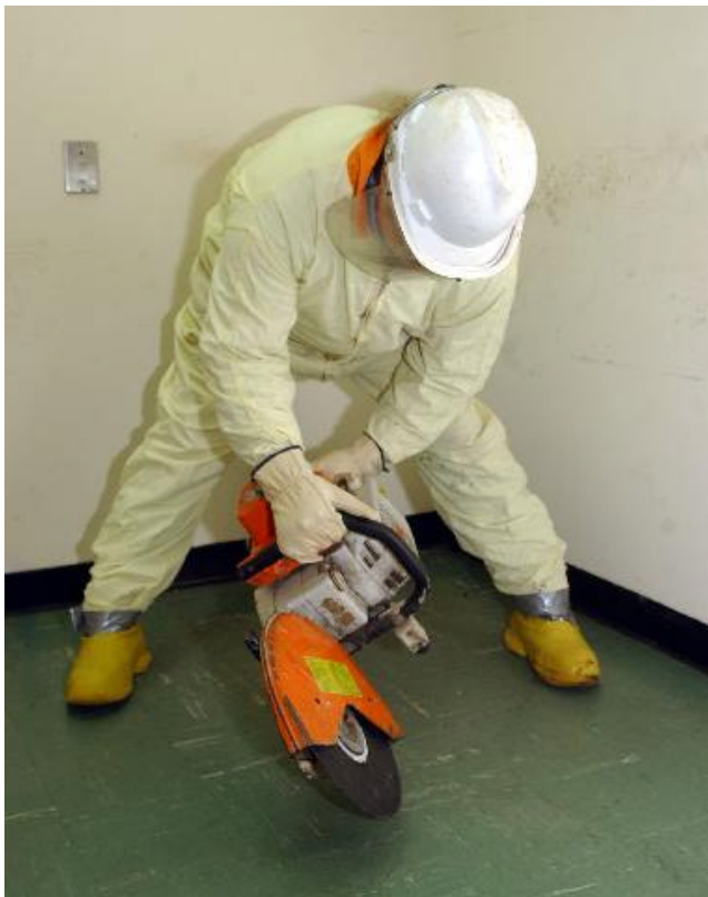
Figure 10. Laborer Demonstrating Use of Cut-Off Machine (Held in Incorrect Position)
