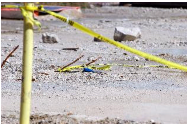
Figure 2. Closeup of Rebar at K-1302 Pad
