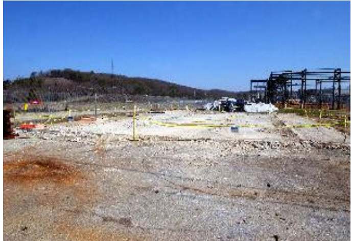
Figure 1. K-1302 Pad at ETTP
