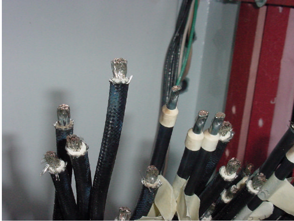
Exhibit 12. Wire With Crimping Sleeves and Without
