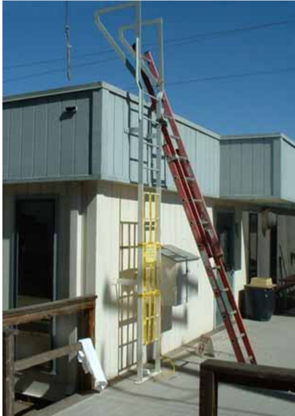
Figure 1.2-1: The scene of the accident. The extension ladder was added after the accident to provide temporary roof access. Barely visible on the right side of the fixed ladder is the rope that the worker used to lift his tool bag onto the roof.
