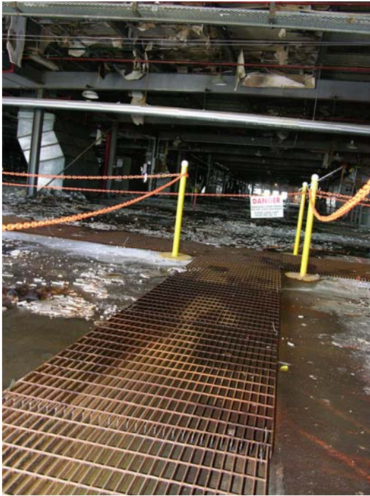
Figure 2-1. Grating walkway on the operating floor.
