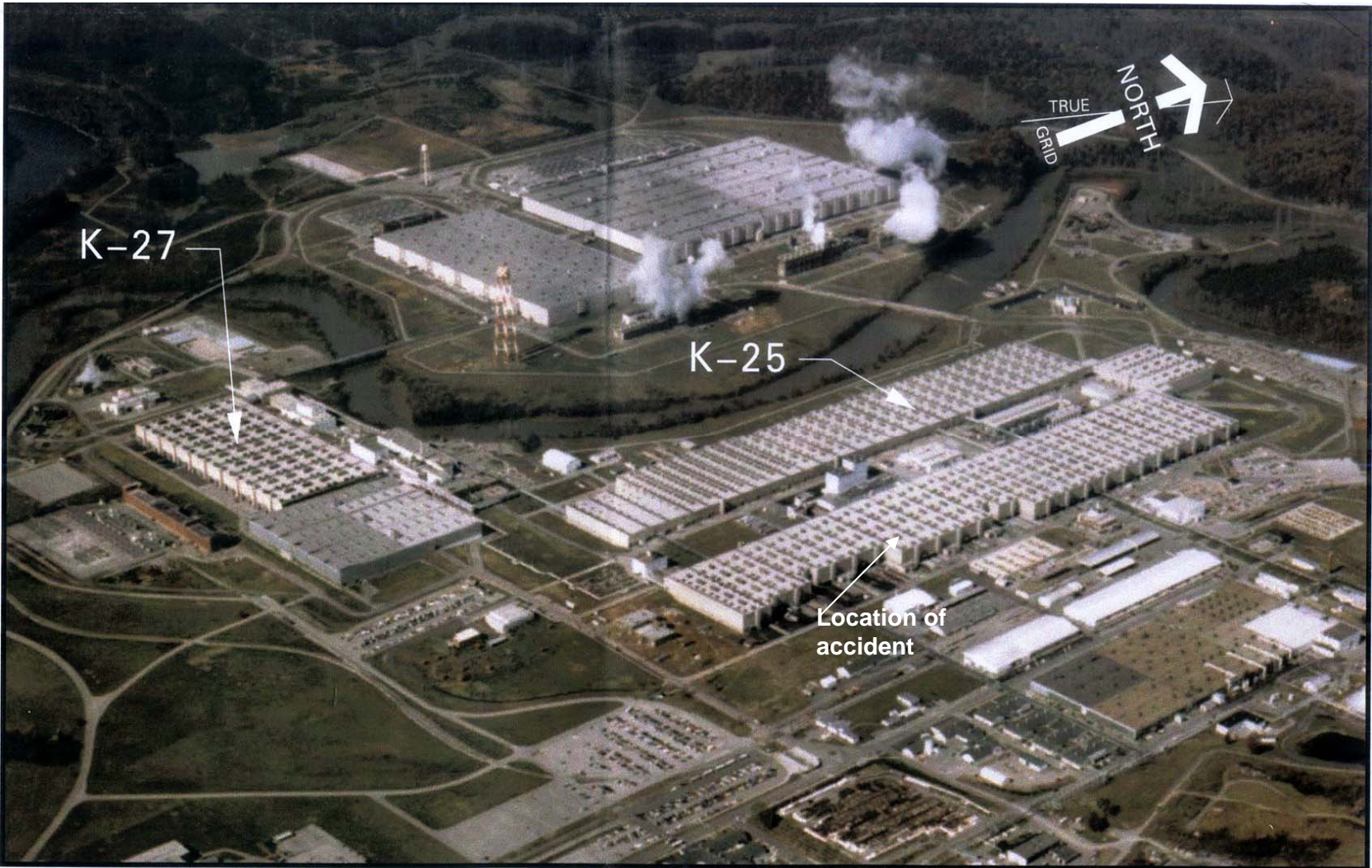
Figure 1-1. Aerial view of the K-25 and K-27 Buildings and the location of the accident
