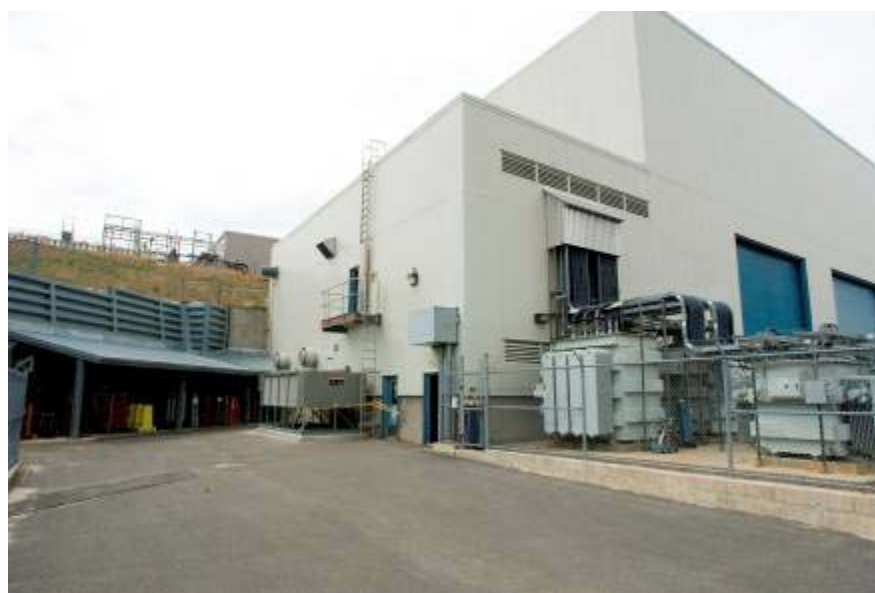
Figure 1-2. Building 1006A (Arc flash occurred in the Mechanical Equipment Loft on the east side of the building)
