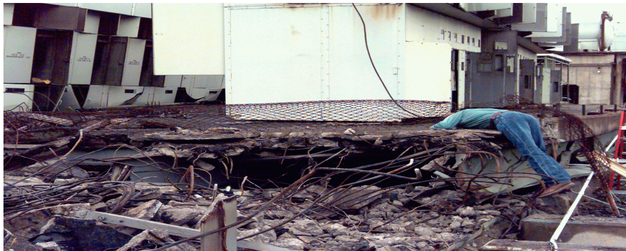
Exhibit 2-5. View of Accident Scene with Simulation of Ironworker Apprentice.
