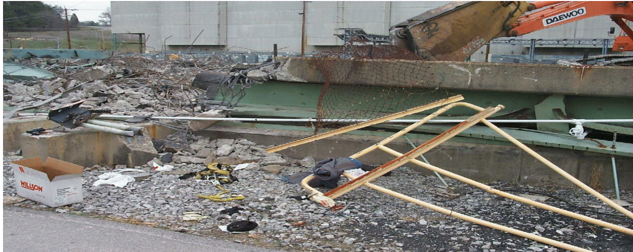
Exhibit 2-4. View of Fence with Attached Railing.
