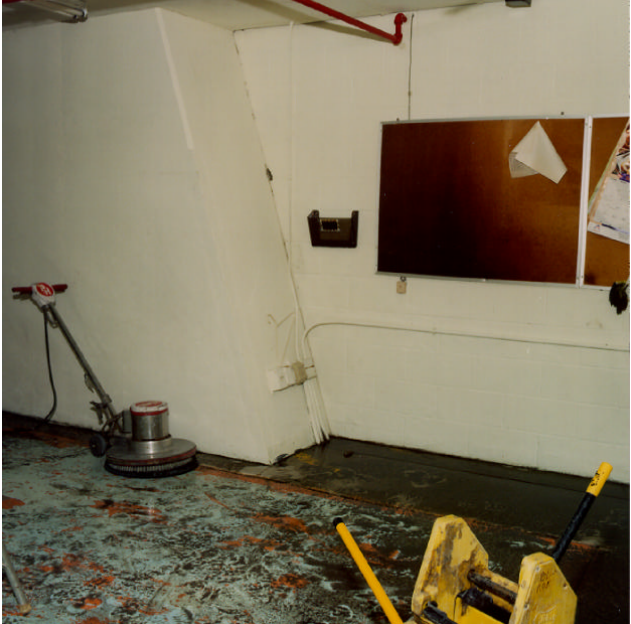
FIGURE 4 Photograph of the Dry Storage Room after the Accident. When the fire/explosion occurred, Painter A was standing near the yellow mop bucket in the foreground and Painter B was using the floor buffer in the background.
