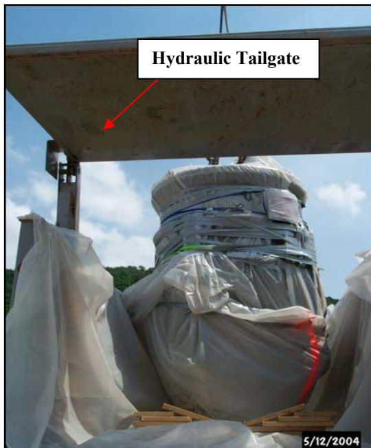
Figure 2-4. Tank T-12 Being Placed into a Truck Bed Lined with Plastic
