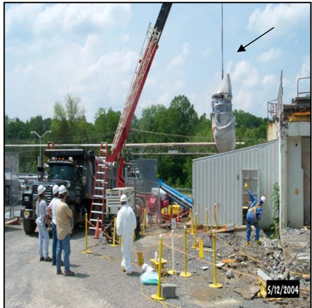
Figure 2-2. Lifting a Tank from the T-13 Annex
