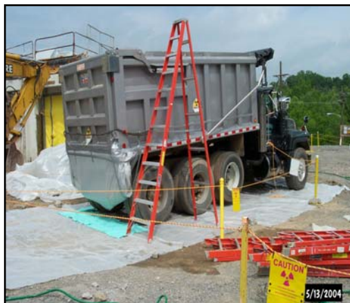
Figure 2-6. Tilting the Truck Bed to Collect Any Additional Liquid
