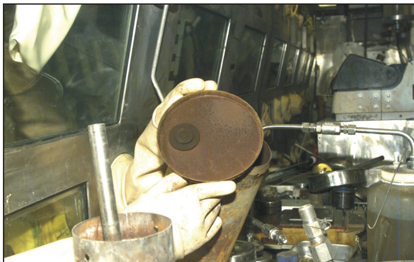
Exhibit 3-1 Acorroding can in a nitric acid glovebox in room 201.
