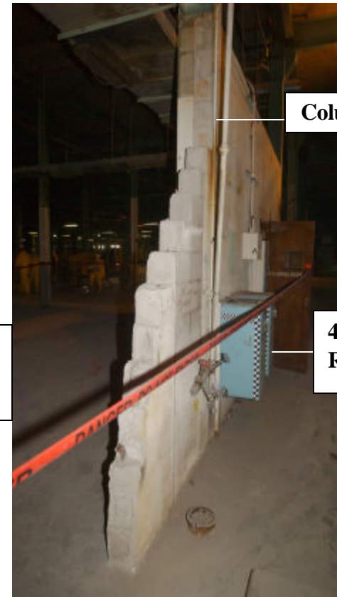
Exhibit 2-6. View of Remaining East Wall of Control Room (Looking North)
