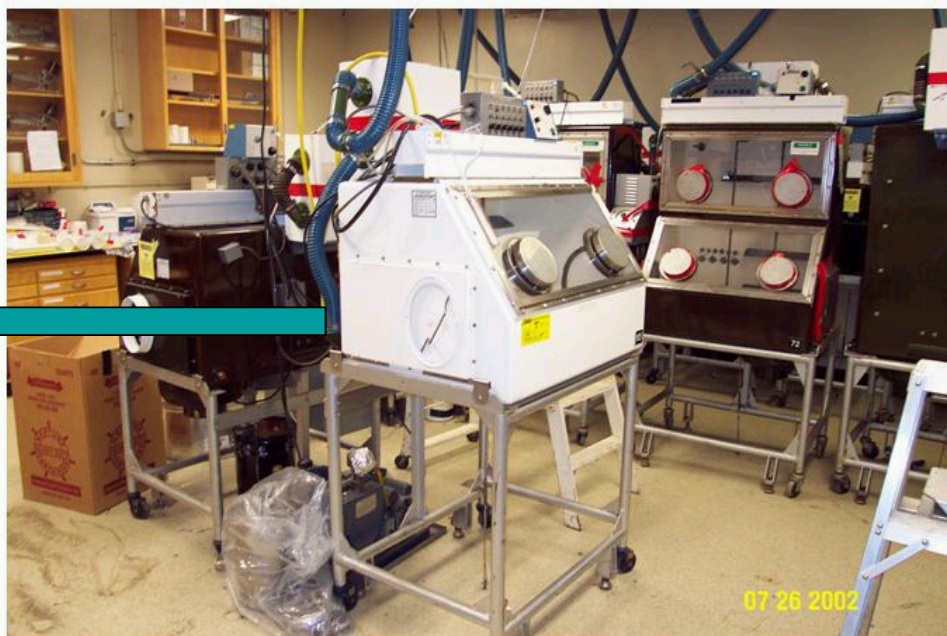
Figure 5. Glovebox 65 in Room “B”.
