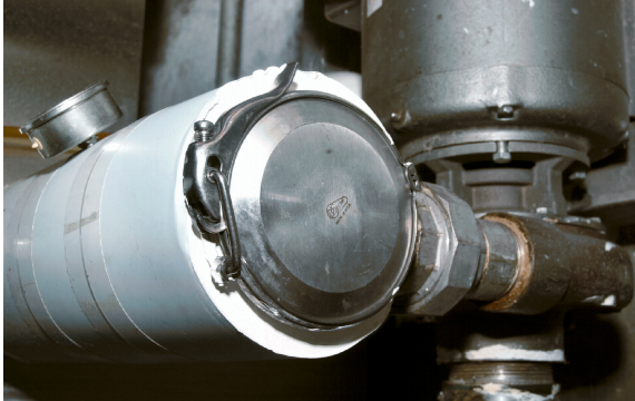
Exhibit 2-2. Latch and Filter Assembly
