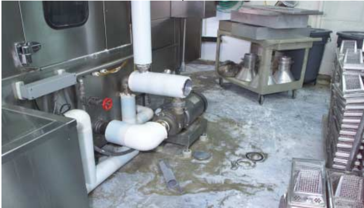
Exhibit 2-4. Hot Water Pipes
