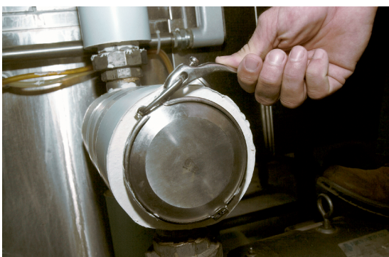
Exhibit 2-3. Filter Assembly Clamp
