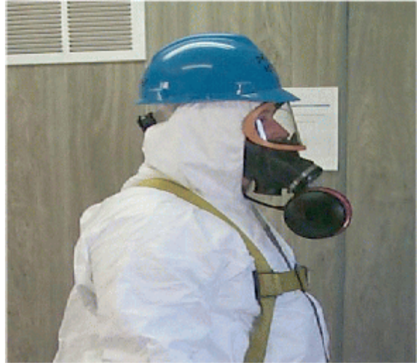
Exhibit 2-5. Asbestos Worker PPE for the MRF D&D Project – Side View
