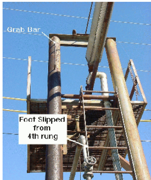
Exhibit 2-10. Closeup View of Top of Ladder
