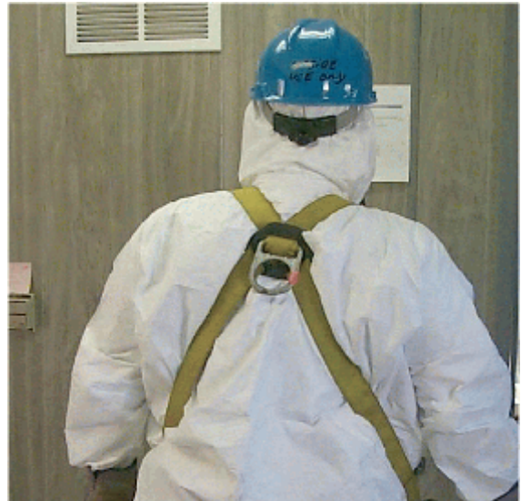
Exhibit 2-6. Asbestos Worker PPE for the MRF D&D Project - Back View
