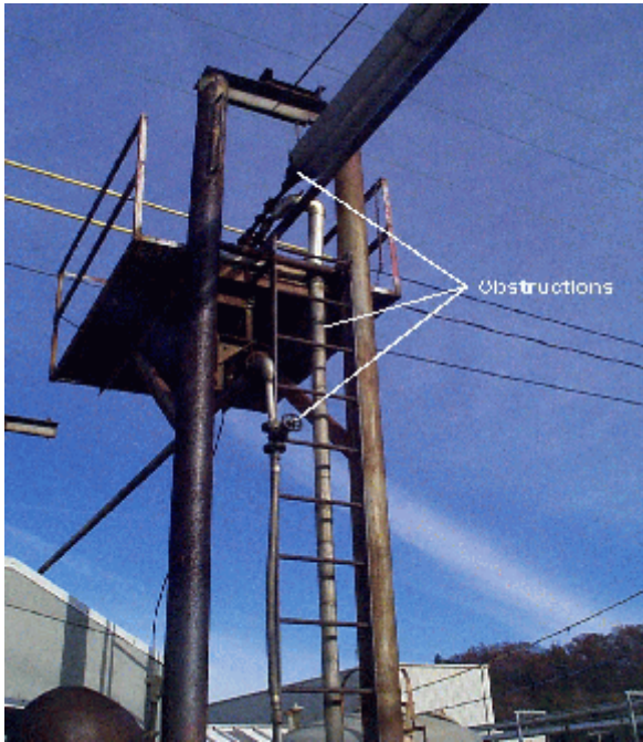
Exhibit 2-9. View of Fixed Ladder with Obstructions
