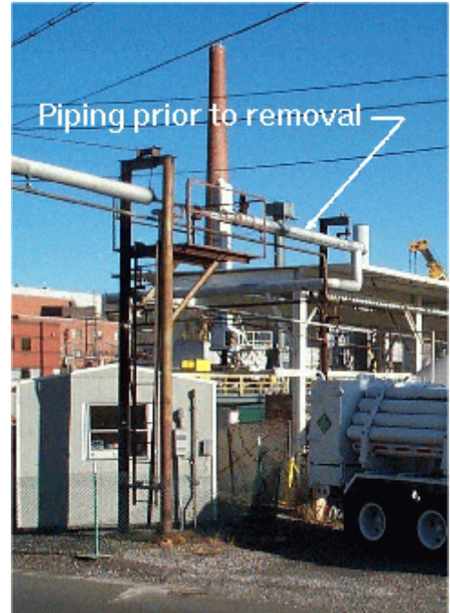
Exhibit 2-1. Work Platform Before Pipe Removal
