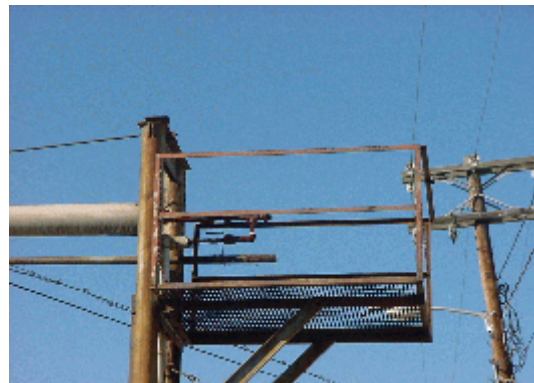
Exhibit 2-2. Work Platform After Pipe Removal
