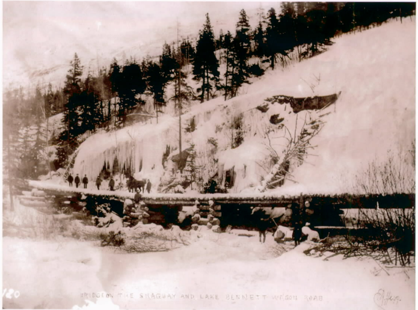
Log Bridge on the White Pass Trail, Alaska, ca. 1898. Photograph by Eric A. Hegg. Courtesy MSCUA, University of Washington Libraries. Negative: Hegg 120
