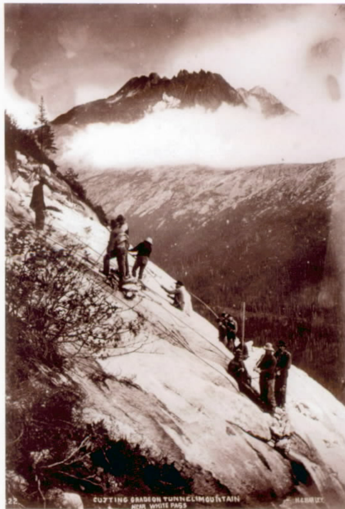
Cutting grade on Tunnel Mountain near White Pass. Photograph by H.C. Barley. Courtesy MSCUA, University of Washington Libraries. Negative: UW 21937
