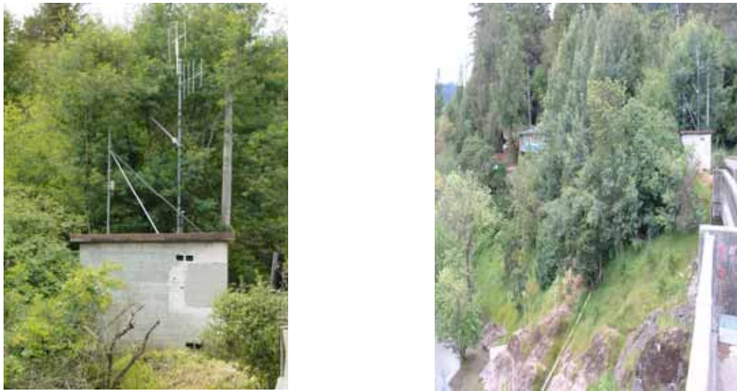
Figure 10. USGS gage 1467000 located on the right bank of the Russian River near Guerneville, CA. taken from the Hacienda Bridge with railing showing in the lower right of each photograph. Details of the telemeter equipment above the gage house is shown in the left image. In the right image, the instrumentation conduit is seen running down the bank into the river.
