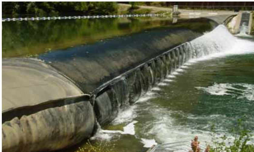
Figure 4. The inflatable dam is constructed of 'automotive-tire' type rubber and is inflated with water. The fish ladders may be seen on either bank downstream of the dam.
