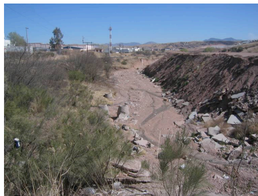
Figure 2. Nogales Wash showing sediment source on right bank and manholes in the channel bottom.
