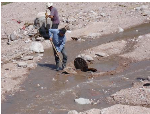
Figure 1. OOMAPAS-NS maintenance crew addressing impacted infrastructure in Nogales Wash.
