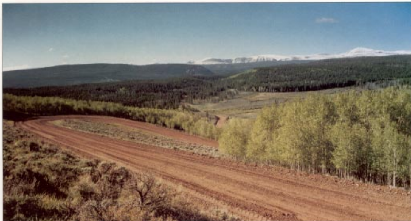
The Loop Road wraps around four oil fields developed by Showcase partners under the multiple-use concept.
