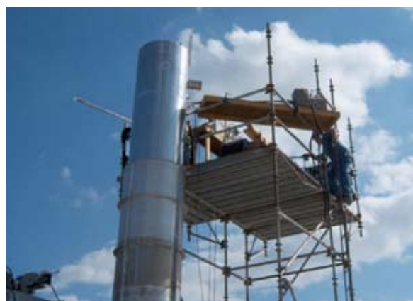
Figure 2-7. Telescoping Stack
