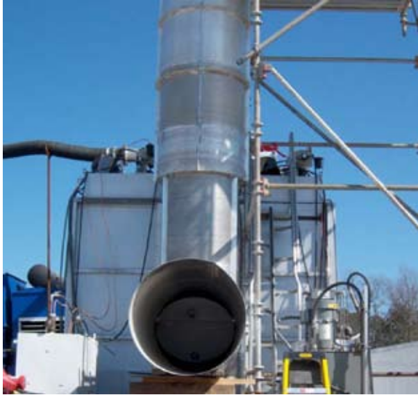
Figure 2-8. Stack Dilution Inlet
