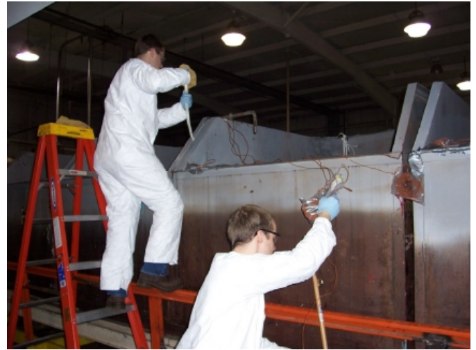
Photo 38. Stringing Thermocouple Wires Along the Top of the Bins
