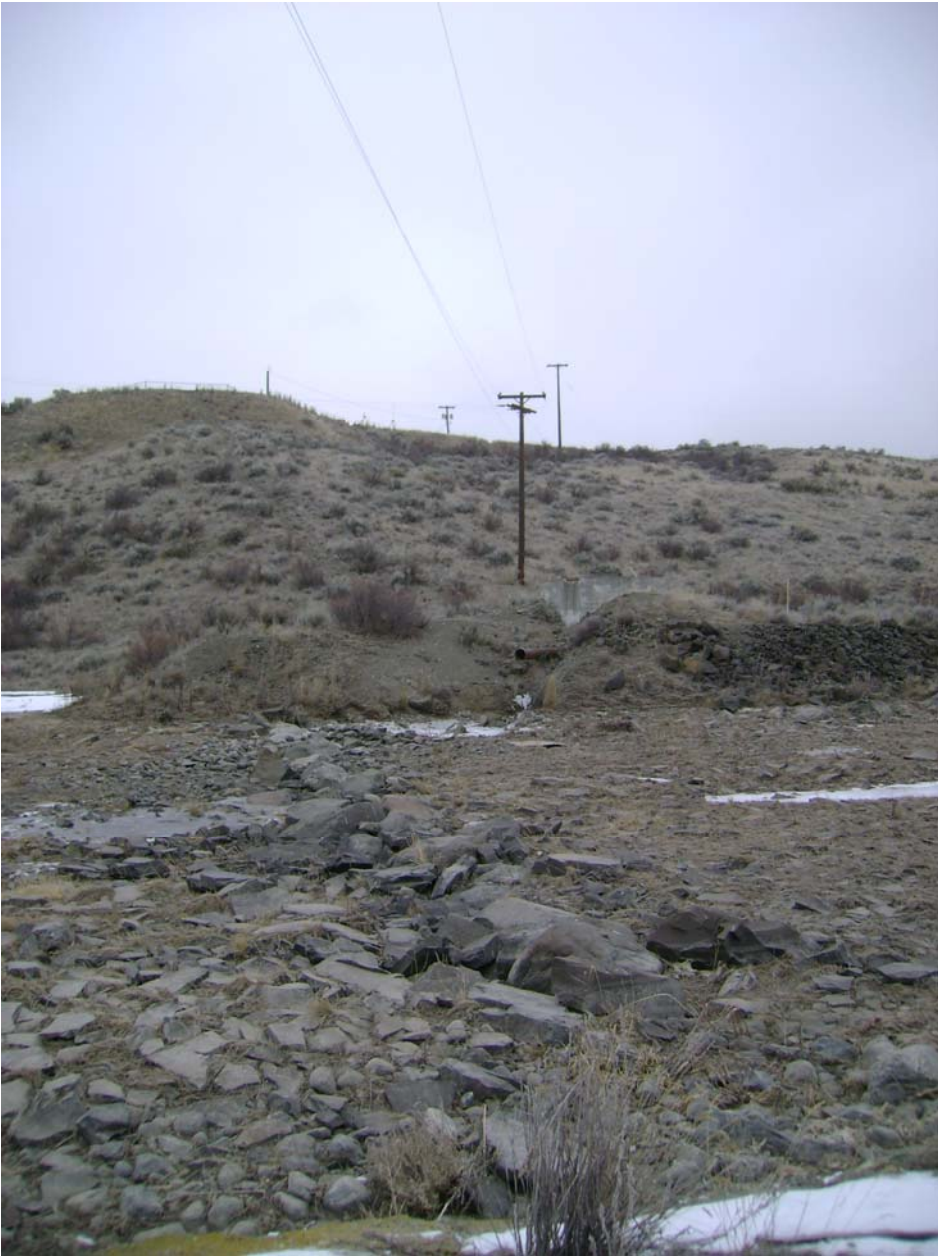
FIGURE E-1 Riprap covering the East-Low Siphon
