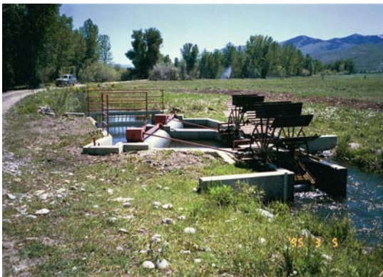
Photo 2.3-4. New fish screen in Lemhi Subbasin.
