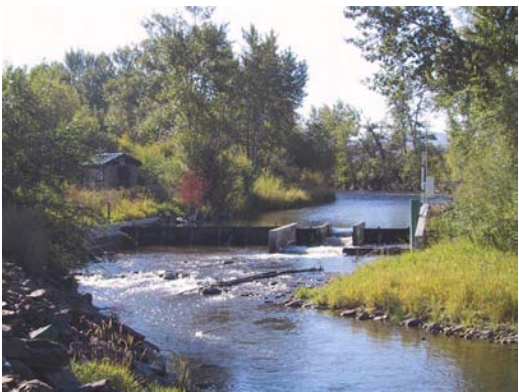
Photo 2.3-1. L6 Diversion structure on the Lemhi River.
