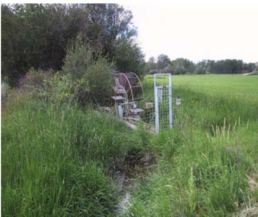
Photo 2.3-5. Nonconforming wiper-style fish screen.
