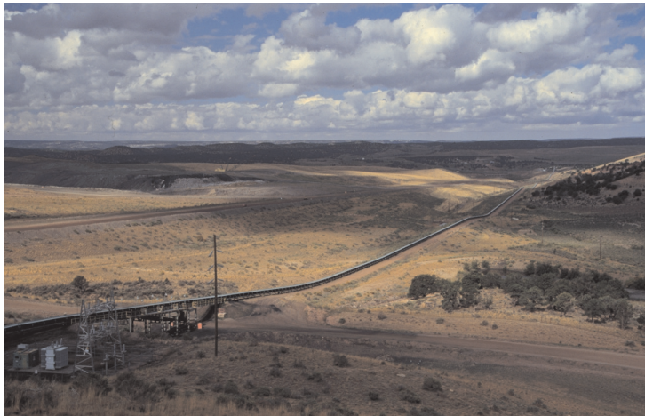
Figure 29B. Part of the 17-mi-long conveyor system from the Kayenta mine to the Black Mesa and Lake Powell Railroad. The belt can transport as much as 1,800 short tons per hour.
