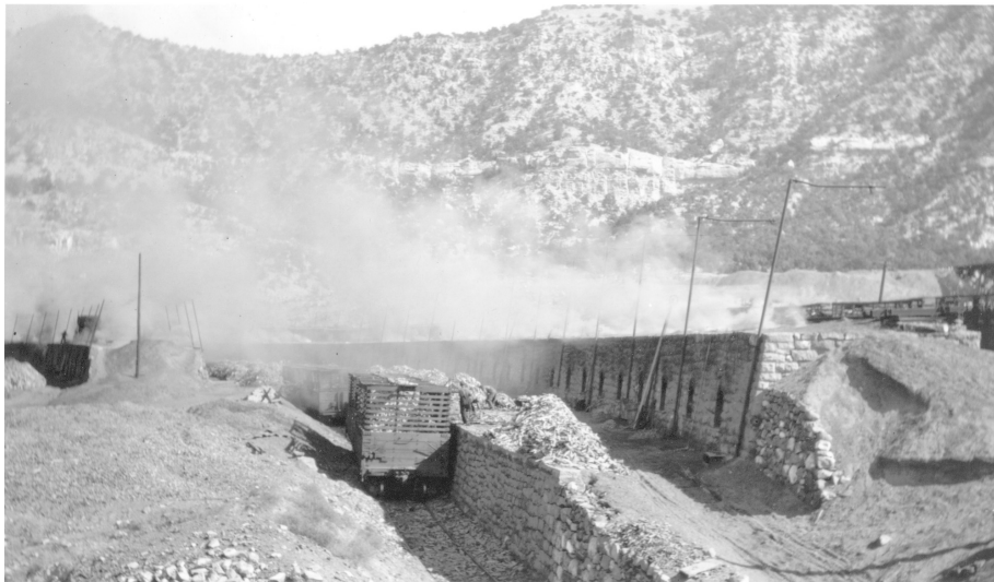
Figure 24A. Sunnyside, Utah, coke ovens, which first operated in 1902 (Clark, 1928). The coke was used in the production of steel.
