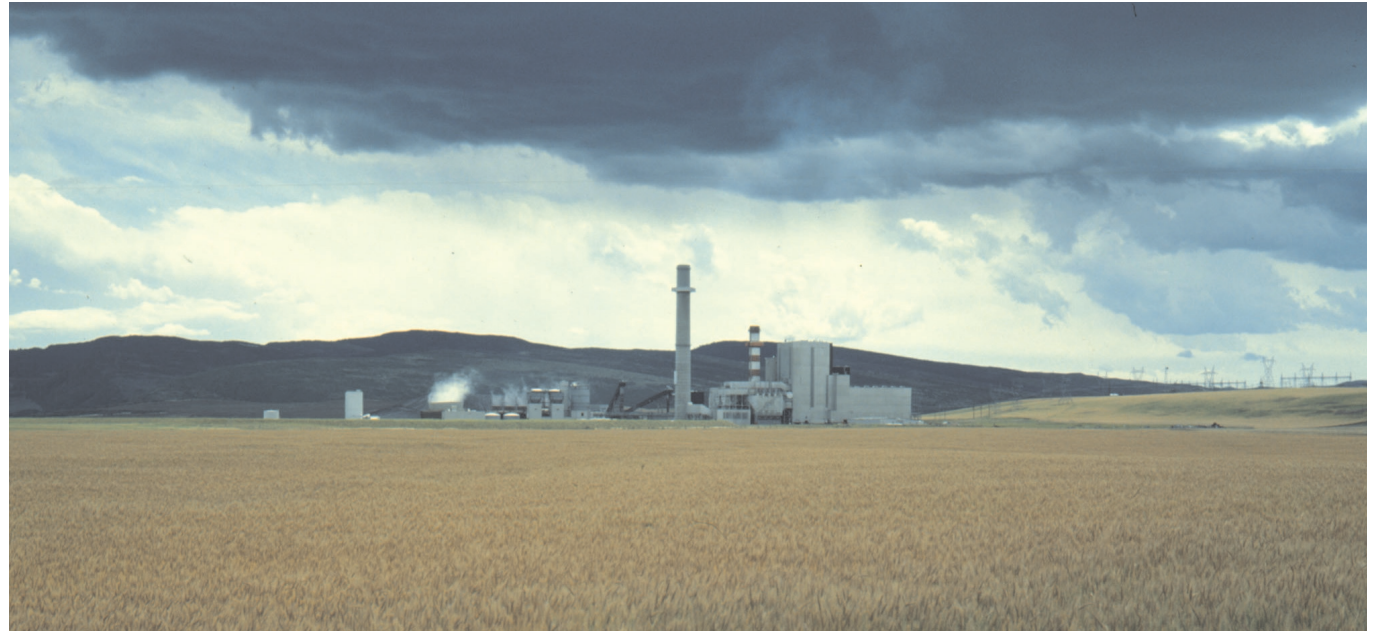
Figure 32A. The Hayden power plant located in northwestern Colorado in the Yampa coal field. Photo by Edward A. Johnson, U.S. Geological Survey.
