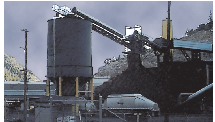
Figure 30. Loadout facility of the Soldier Canyon mine in the Book Cliffs of Utah showing the loading of specialized trucks for transporting coal. Photograph by Russell Dubiel, U.S. Geological Survey.
