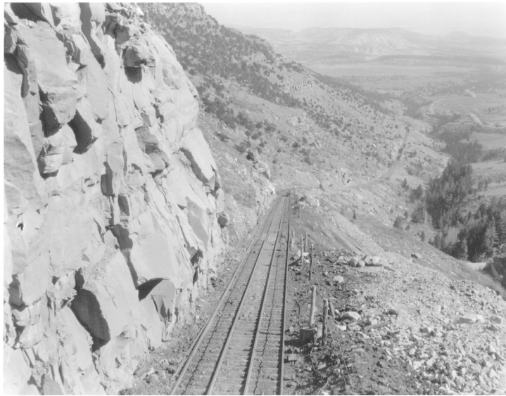
Figure 29A. Tramway system at the Wattis mine in the Wasatch Plateau, Utah (first published by Spieker, 1931, plate 1B). The tramway is 1.25 mi long, had a maximum grade of 36 percent, and could move 10 cars at a time to a tippie that had a capacity of handling 1,500 short tons a day (Spieker, 1931, p. 115). Note the cable running up the length of track that allowed the hoist to pull the cars up the incline.
