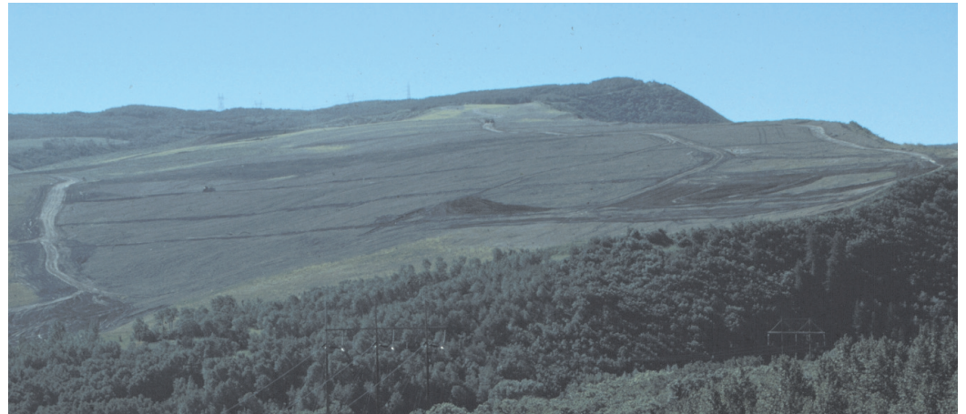
Figure 33. Edna mine in the Yampa coal field of Colorado being reclaimed during 1995.
