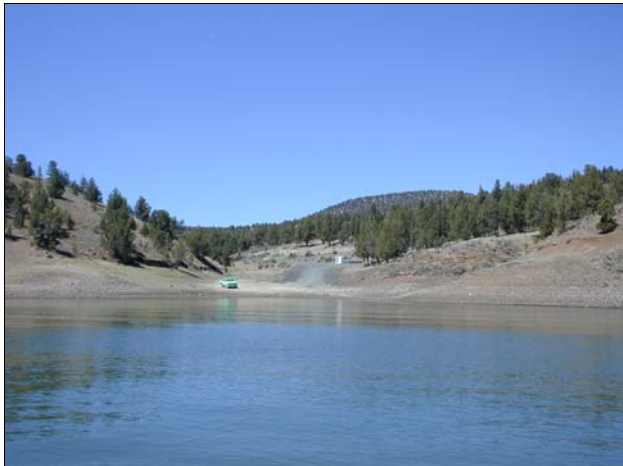
Photo 3-14. County Boat Ramp.
