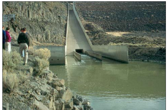
Photo 3-1. Bowman Dam spillway.
