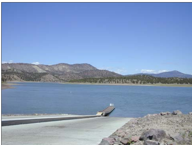
Photo 3-4. State Park boat ramp.
