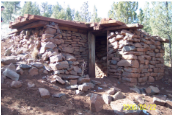
Photograph 10. Stone structure, believed to be the powder house.
