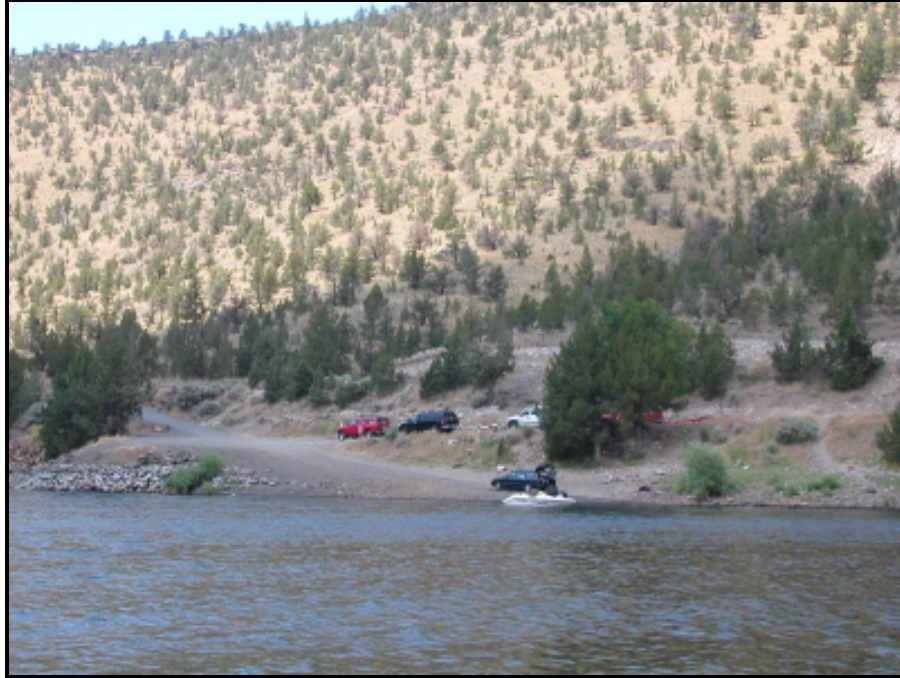
Photograph 4. Existing ramp and parking.
