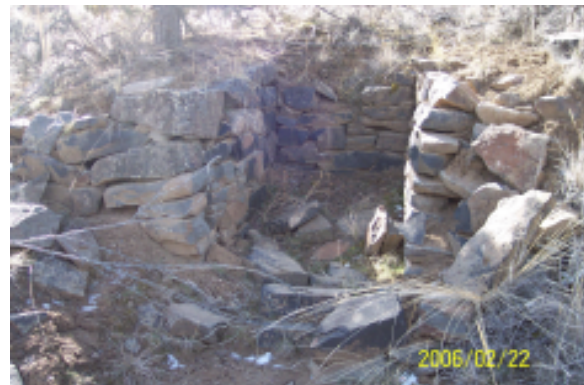
Photograph 11. Separate small structure, possibly for storing blasting caps.
