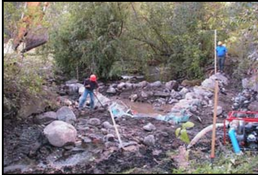
Photo A-21. Looking downstream at Weir No. 3 just prior to completion. The worker at center-left is filling the spaces between the large rocks with cobble-size material and fines.
