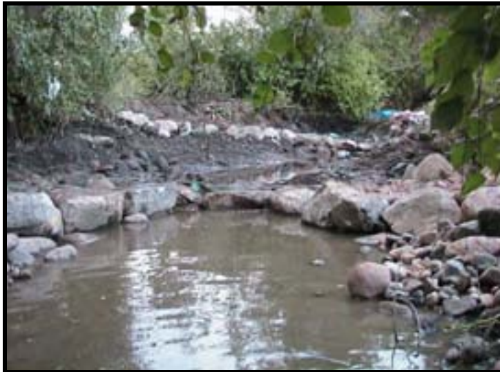
Photo A-23. Looking upstream at the lower weirs (Nos. 3 and 2).
