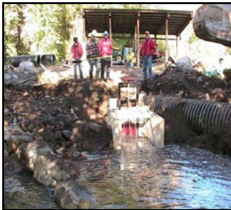
Photo A-14. The newly installed diversion box was tested and satisfied the flow requirement for the landowner's water right.
