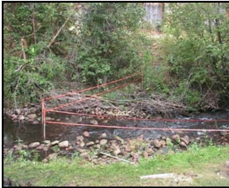
Photo A-2. Preliminary layout of upper weir (Weir No. 1); flow is from left to right.
