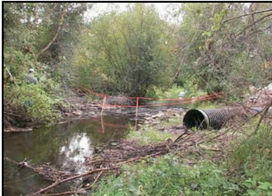
Photo A-4. Looking downstream at entrance to dewatering pipe and the Weir No. 1 layout. The cofferdam will be located between the pipe and the layout.
