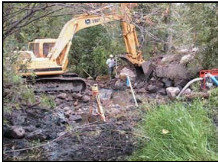
Photo A-20. Looking downstream at initial excavation of Weir No. 3. The concrete at right of photo is the upstream wall of the former diversion dam. The wall and the dam were about the same height (as shown in Photo A-1).
