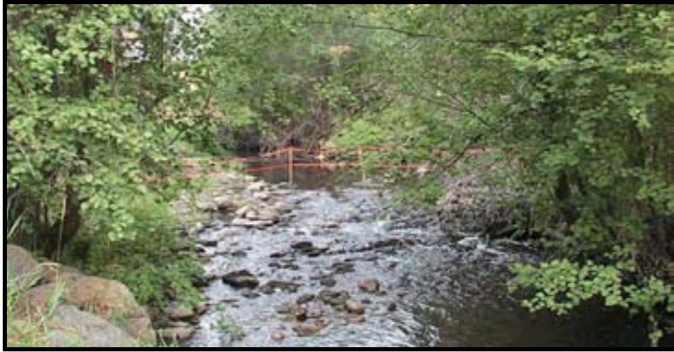
Photo A-3. Looking upstream at Weir No. 1 showing the drop to pool. The height of the riffle ( \pm 10 inches) equals the amount of headloss available to deliver the irrigation water.
