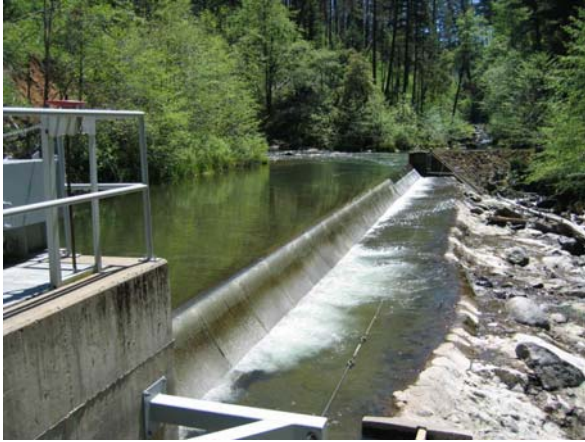
Figure A-1. Montgomery Creek intake.
