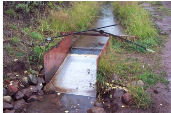
Figure A-4. A small Coanda-effect screen provides water to a sprinkler irrigation system near Carbondale, Colorado.
