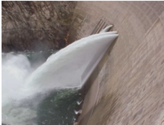
Figure 1. - Arrowrock Dam: Operation of existing outlet works.
