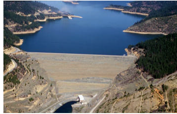
Figure 1. — Trinity Dam and Reservoir, Central Valley Project - California.
