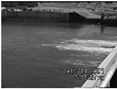
View of white water turbulence downstream of gates 5, 6 and 7.
