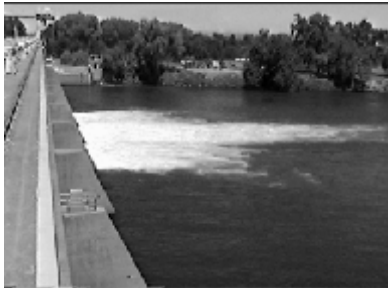
View of white water turbulence downstream of gates 5, 6 and 7. Surface turbulence extended well downstream of the stilling basin endsill.
