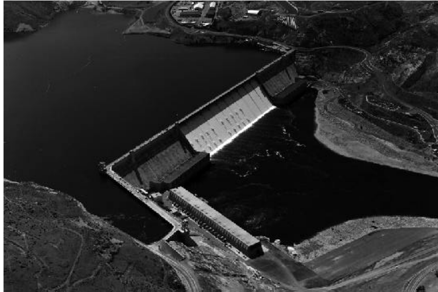
Figure 1. - Overall view of Grand Coulee Dam and Third Powerplant.
