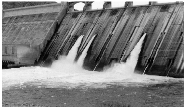
Grand Coulee Dam with mid- and lower-level outlet works operating above and below each other.
