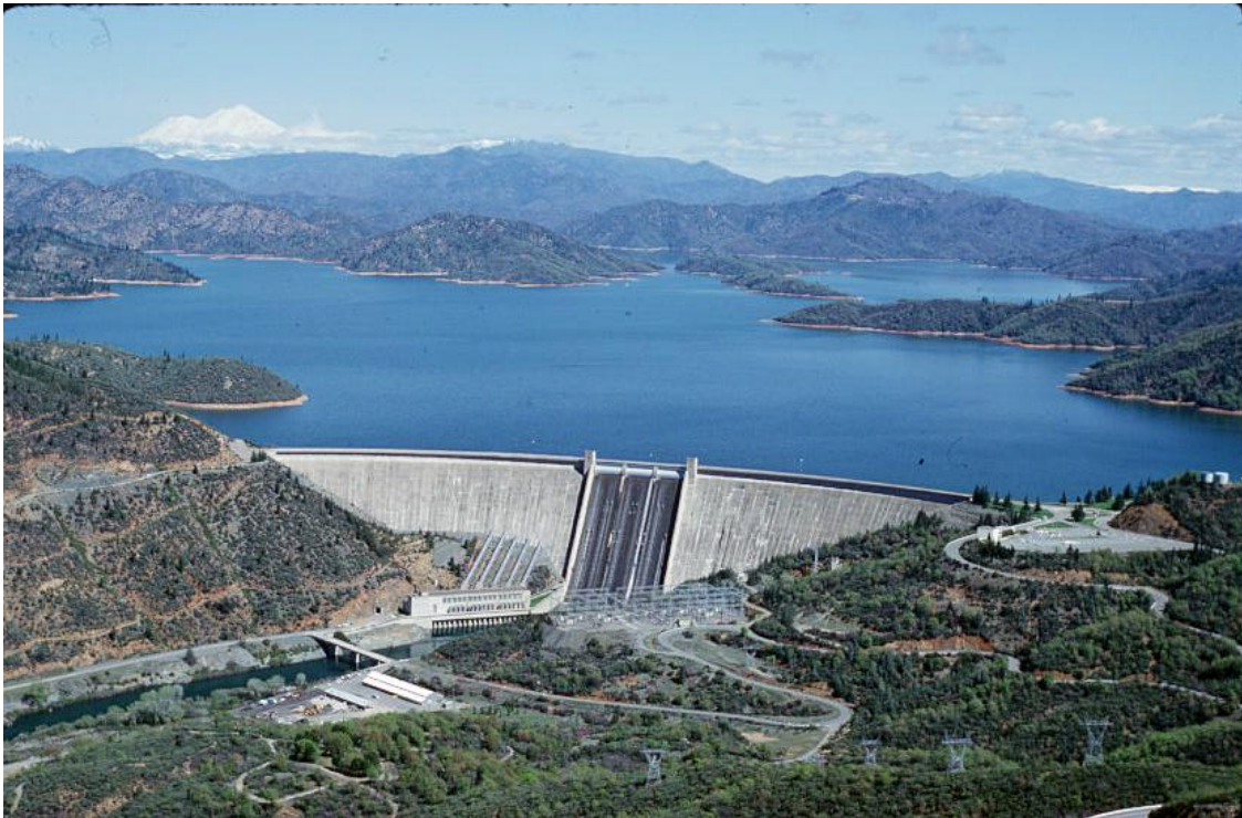
Figure 1. Shasta Dam with penstocks, powerplant, and spillway in the foreground, and Shasta Lake in the background.
