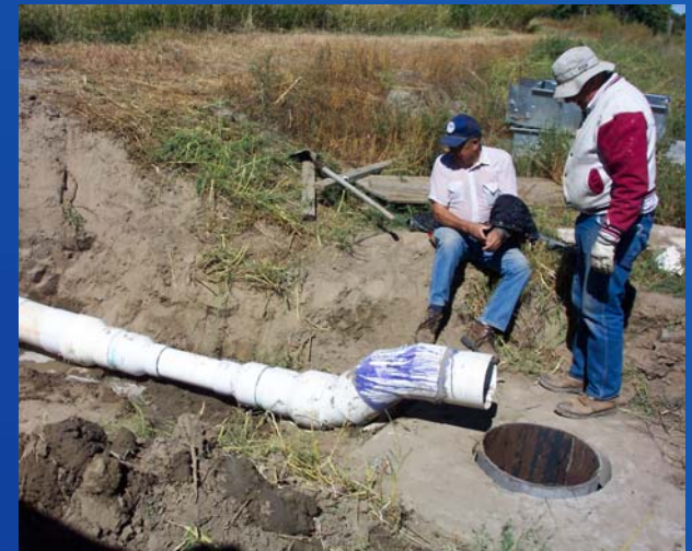
Venturi Meter Made from PVC Fittings
