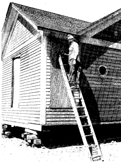
Preparing the Itjen House for painting, 1980.
