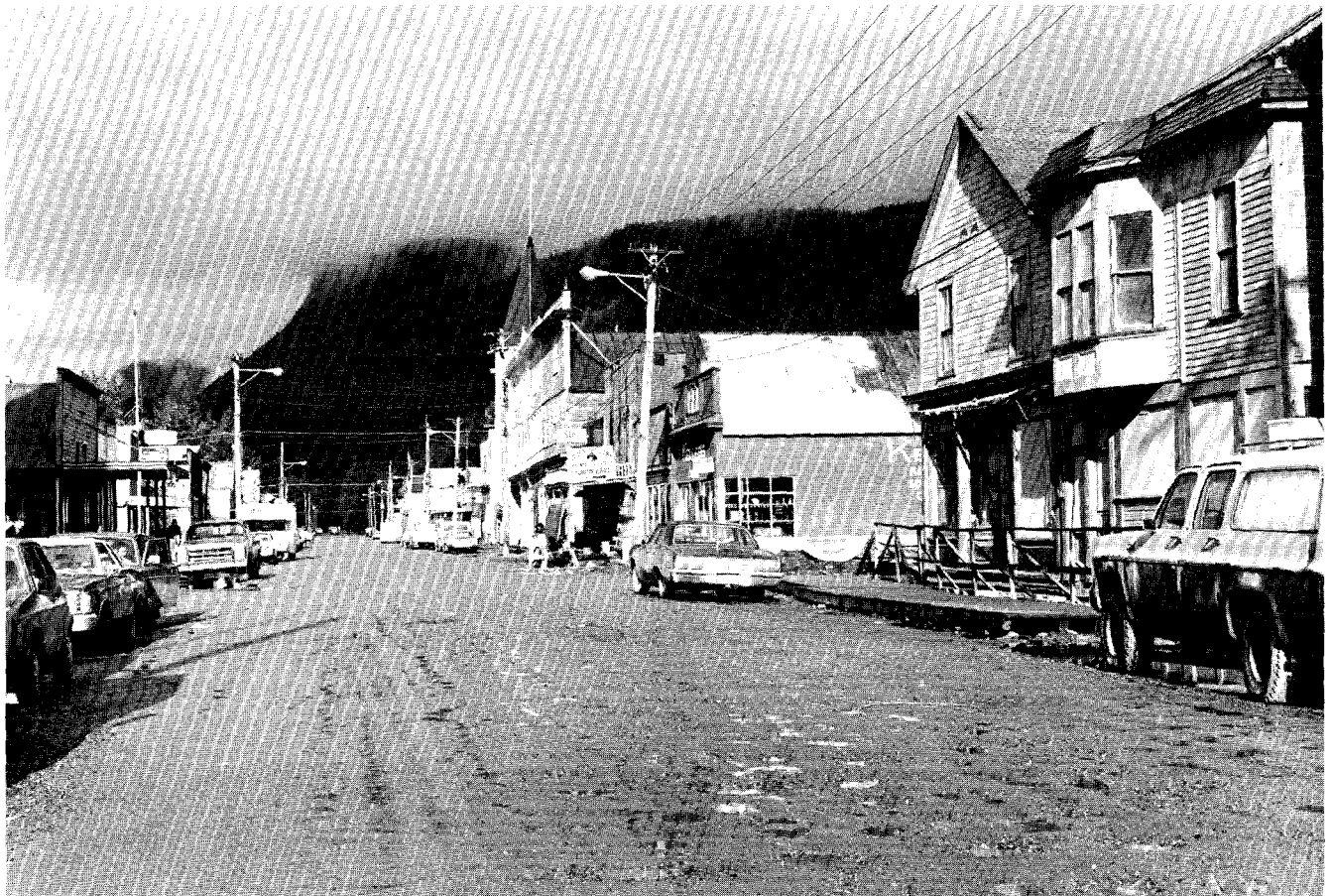
Broadway Avenue in 1979. Restoration of Mascot Saloon underway at right. (Meg Jensen photo)
