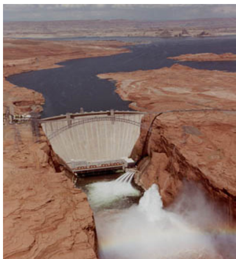
Figure 7. Aerial view of Glen Canyon Dam showing the jet-tubes and the spillways in use.
