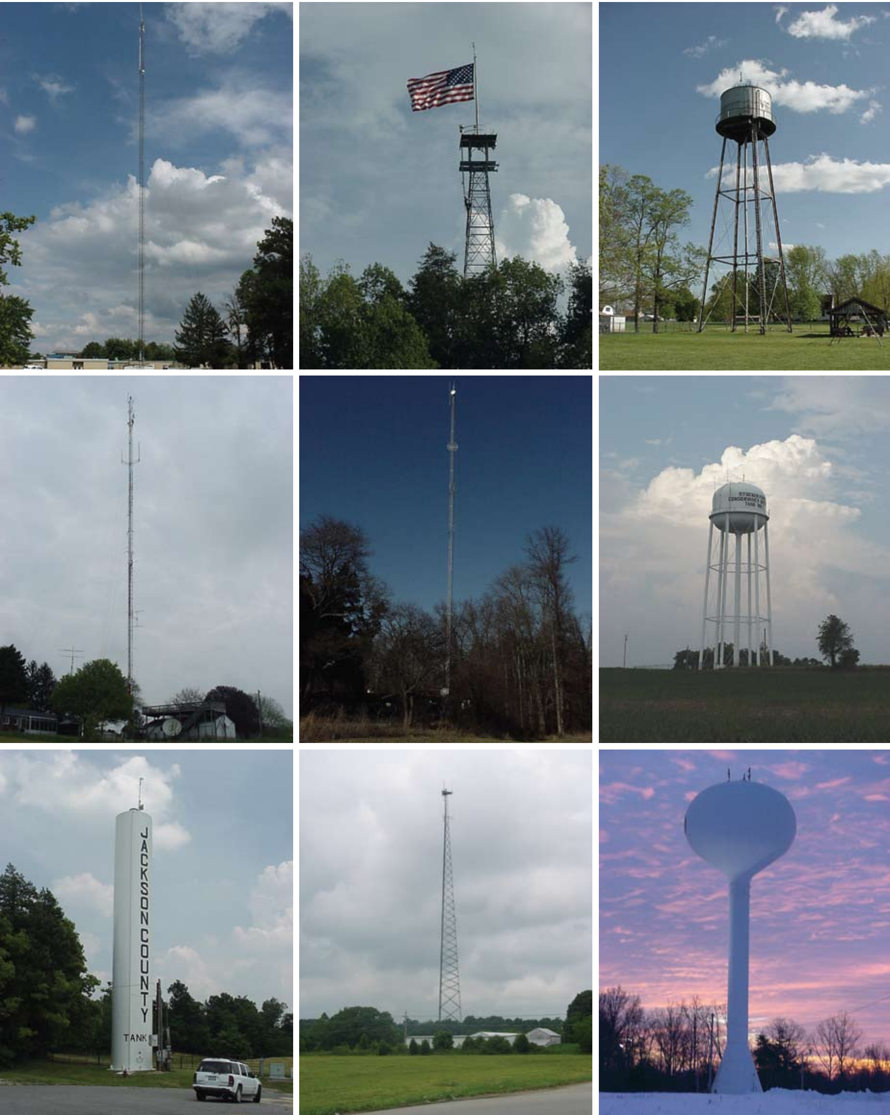
Scottsburg Electric deployed a broadband network using satellite dishes and antenna located on towers throughout the county. By utilizing orthophotography, the utility was able to align the dishes precisely to achieve the best signal.
