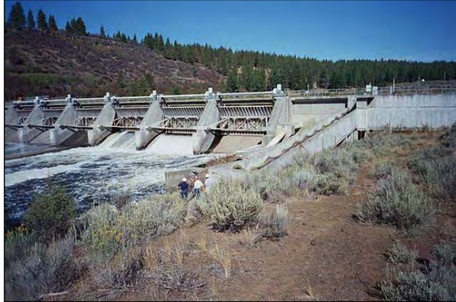
Keno Dam (River Mile 230) is a non-hydroelectric facility and is not part of Reclamation's Klamath Project. The fish ladder facility is visible on the right and is located on the left bank of the Klamath River (looking downstream).
