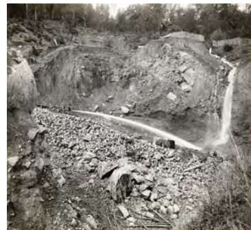
A past gold mine operation within the Klamath River Basin showing hydraulic mining. Unknown date.
