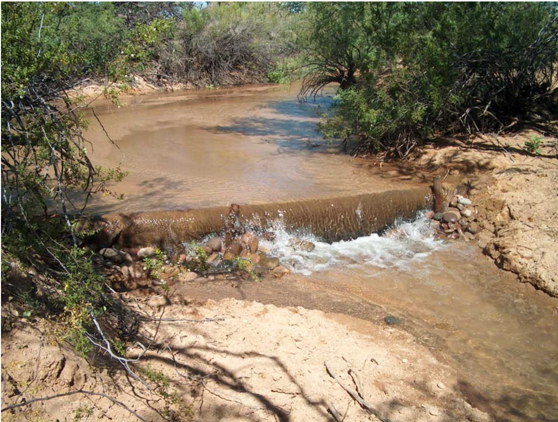
Figure 4. Check dam on Arroyo 19.
