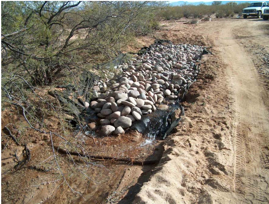
Figure 3. Discharge structure on Arroyo 19.
