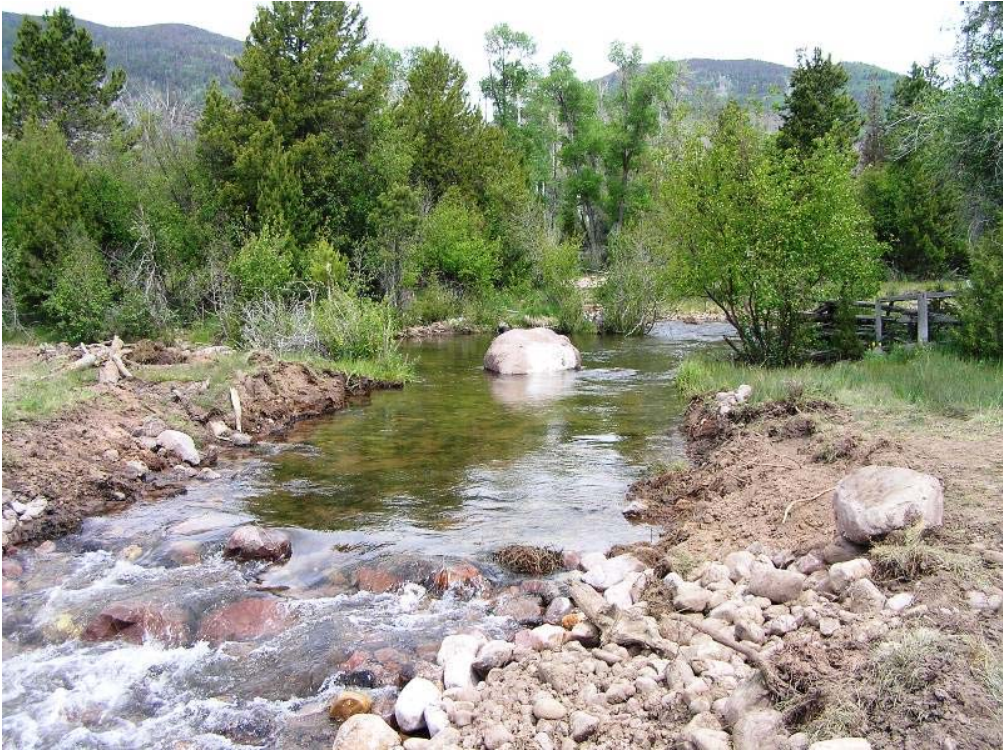
Figure 38, June 11, 2007, newly constructed inlet to “Arrowhead Creek” looking north.
