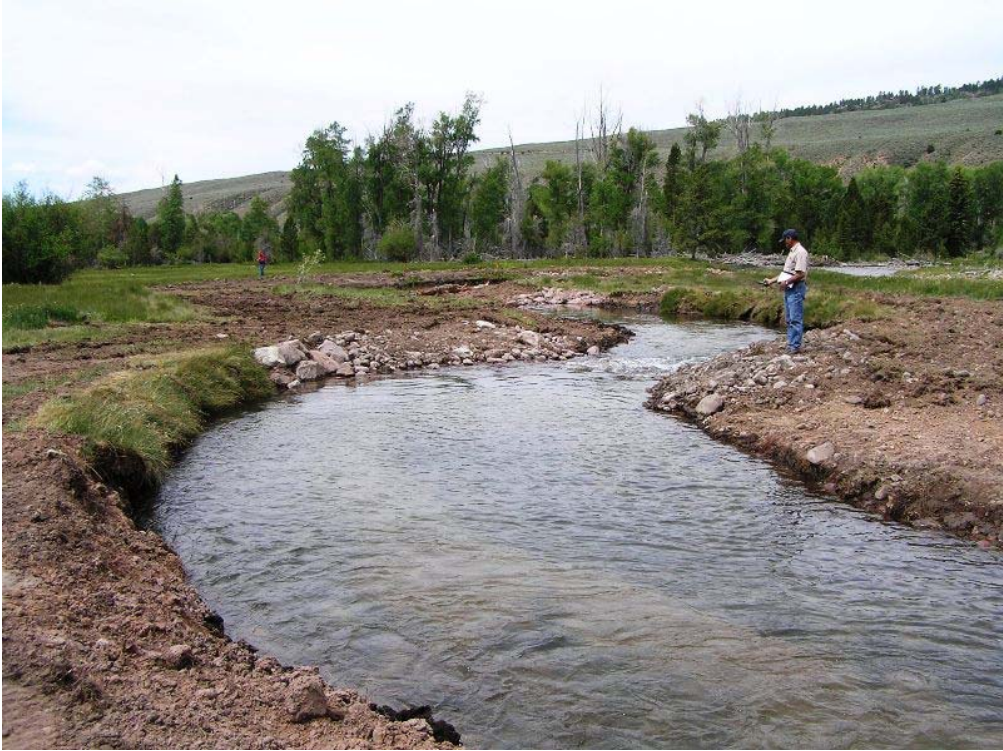
Figure 39, June 11, 2007, newly constructed “Arrowhead Creek” looking SSW.
