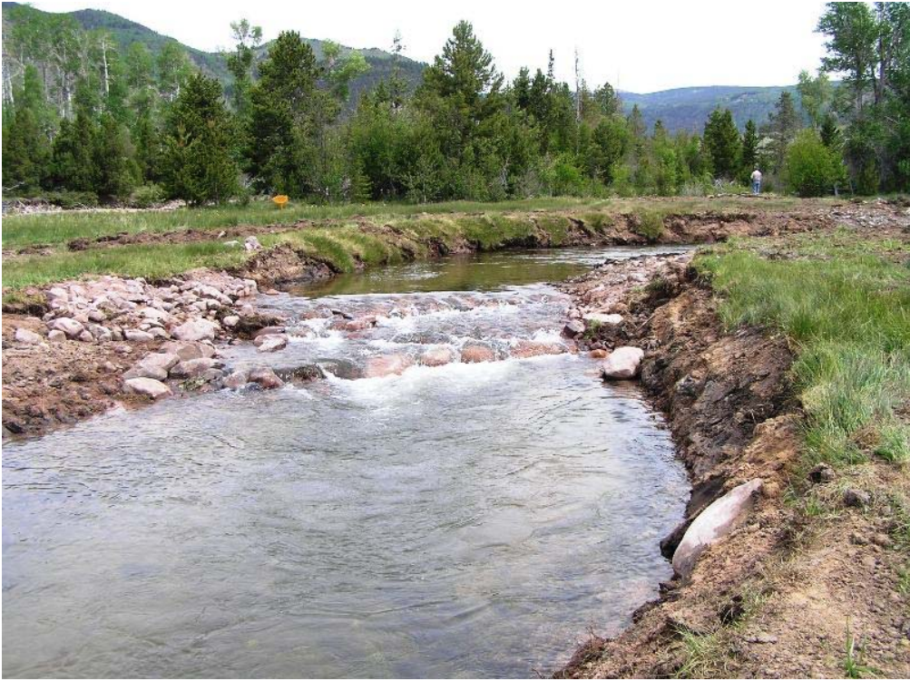
Figure 41, June 11, 2007, “riffle, pool, run” strategy.
