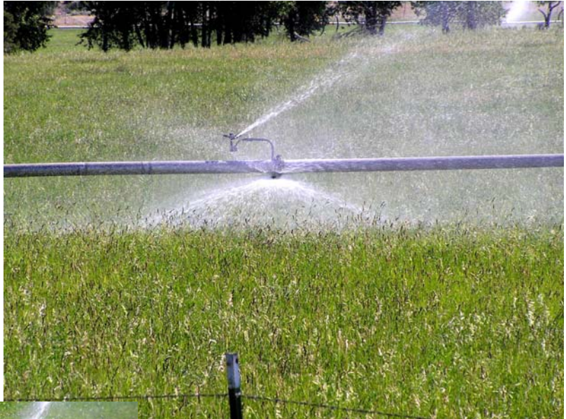
Figure 25, Drain leaks are the most common type of leak – and the most prolific
