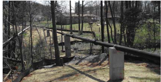
First-time sewer installation for 51 homes in West End Community stops septic tanks from overflowing and creating a stream of sewage that threaten drinking water. Project was funded by a million dollar block grant and City of Mebane matching funds in 2008.
