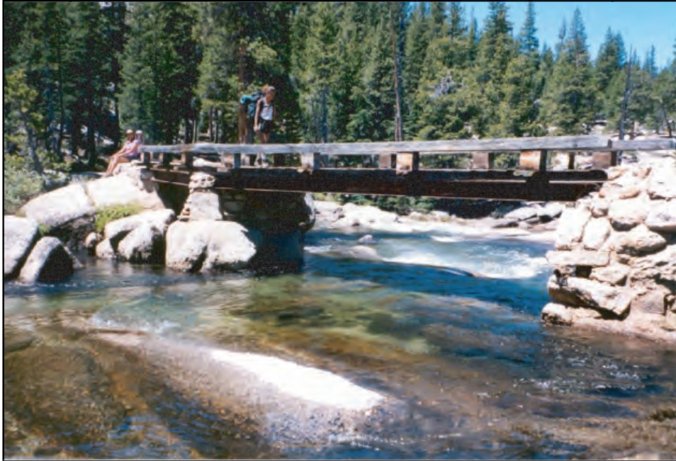
Figure 20: Site 11: Bridge across Tuolumne River above Tuolumne Falls. This will be a standard bridge installation.
