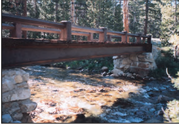
Figure 15 (left): Site 7: Bridge, Dana Fork of Tuolumne River. This will be a standard bridge installation.
