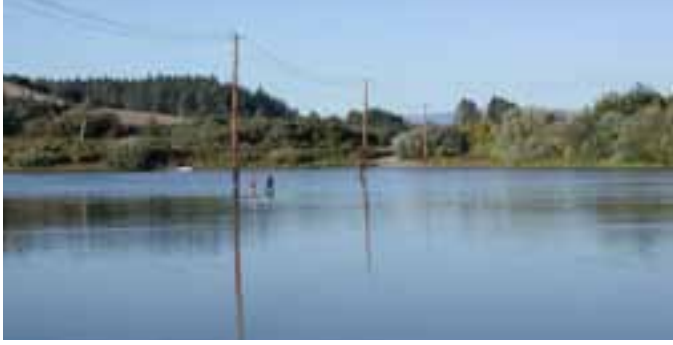
Figure 2. A recharge pond constructed between the Russian River and Westside Road. Power poles extending from supply wells through the ponds toward the road provide scale. Each recharge pond is operated through a cycle in which river water is diverted to the pond for a week or so, then the pond is allowed to go dry for as long as a month to retard the buildup of a clogging algal mat on the pond bottom.
