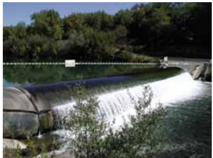
Figure 3. Inflatable dams are constructed of thick rubber for inflation with water for seasonal operation. This inflatable dam has fish ladders on either side to aid in fish migration that may occur during the seasonal operation of the dam. Portage for canoes and other small boats is initiated upstream of white float line.
