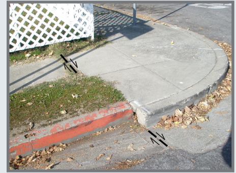
Creep on the Hayward Fault has broken and offset this curb in the city of Hayward.
