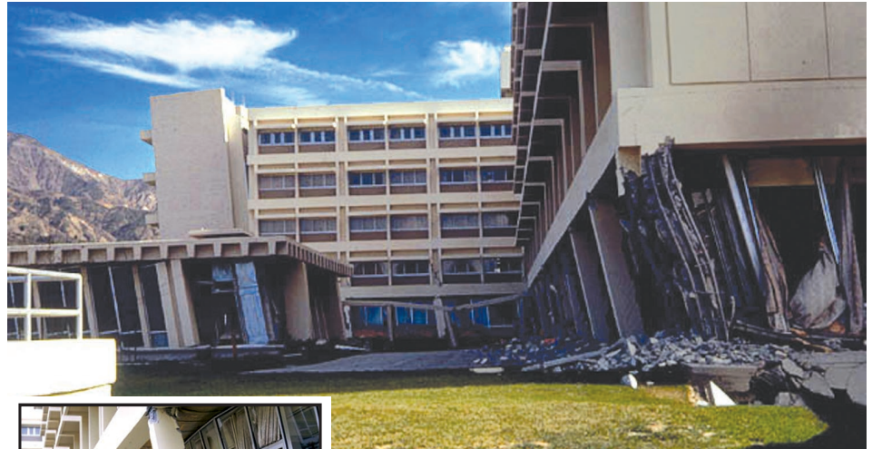
The 1971 San Fernando, California, earthquake (magnitude 6.7) severely damaged the recently built Olive View Hospital. This building was not instrumented with seismic sensors. Accordingly, no data were obtained to understand how the damage initiated and progressed during the intense shaking. The building was razed and replaced with a stronger structure that survived the 1994 Northridge earthquake (see back page).
