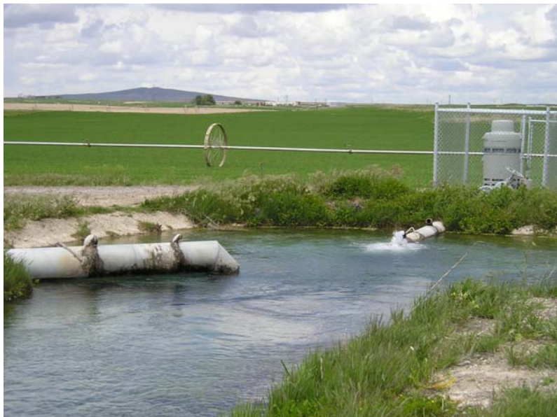
Left: High-capacity well pumping into an irrigation transmission canal on the Snake River Plain, Idaho. In the background is a spray-irrigation "wheel line".
