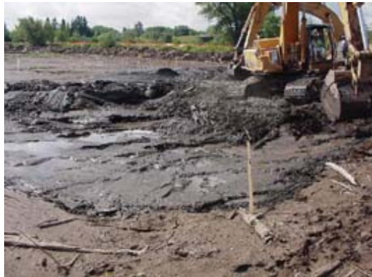
Close-up view of the contaminated sediments being removed from Hog Island Inlet.
