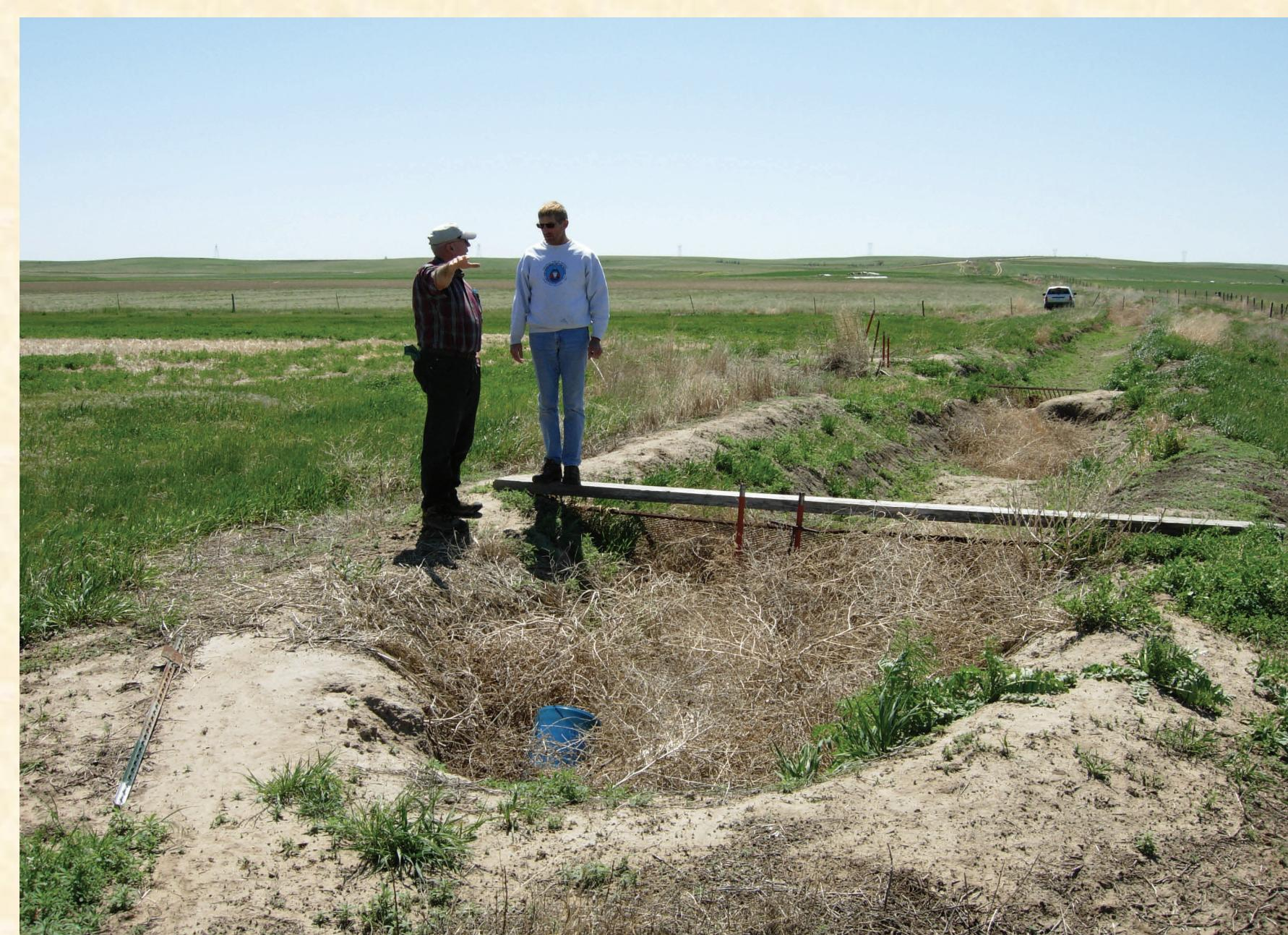
In the fall of 2007 Lateral 18.4 was converted from open ditch to underground pipe. This project was estimated in 2001 to save 90 acre-feet of water per year.
