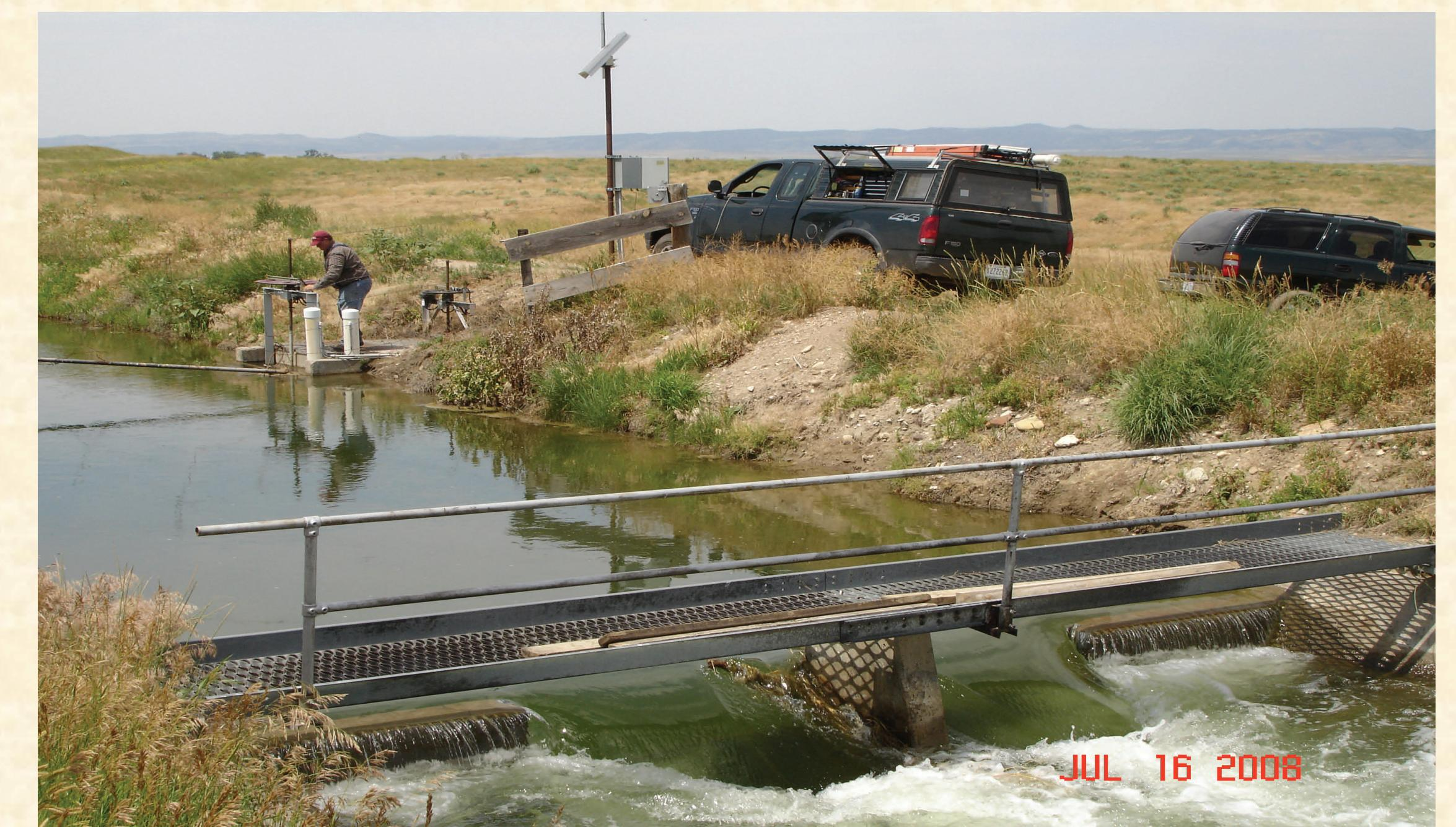
Angostura Irrigation District continues to improve water delivery system efficiency through the installation of automated gate control for laterals.
