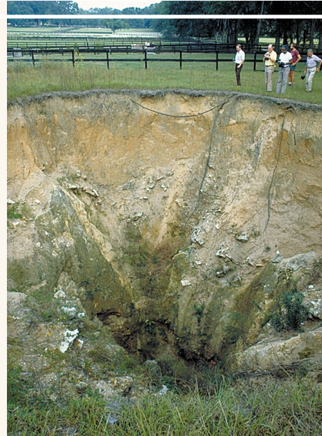
Cover-collapse sinkhole near Ocala, Florida
