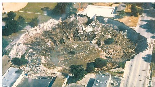
Cover-collapse sinkhole Winter Park, 1981
