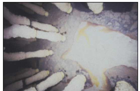
Salt waste is dissolved in the liquid portion of the waste. It can be in normal solution as Supernate (top picture) or, after evaporation, as salt cake (bottom picture) or concentrated supernate. The pipes in all the pictures are cooling coils.
