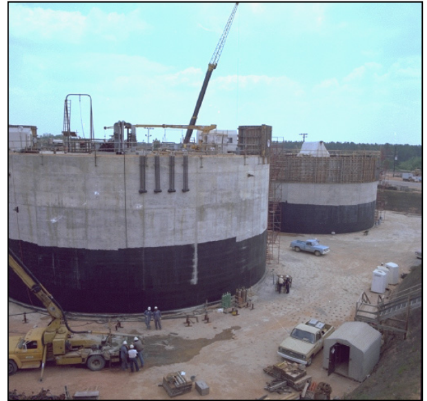
Tanks under construction. Note tank size relative to construction workers. Later, dirt is backfilled around the tanks to provide shielding.
