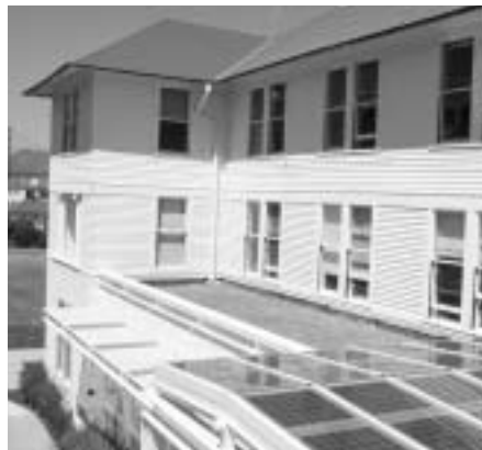
A photovoltaic system over the entryway to this building in San Francisco generates power on site.
