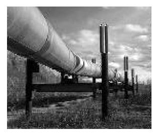
Figure 8: For much of its length, the Trans-Alaska Pipeline is elevated on refrigerated pilings to prevent local thawing and ground instability. Source: ©David Marusek.
