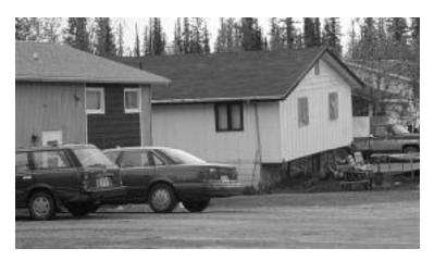
Figure 9: Houses near Fairbanks, Alaska use jacks for support as permafrost thawing causes uneven settling. Source: ©1999, Gary Braasch.
